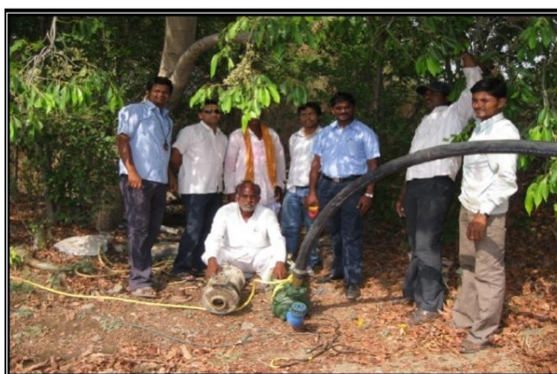
Installation of EE Open well Submersible Pump set
