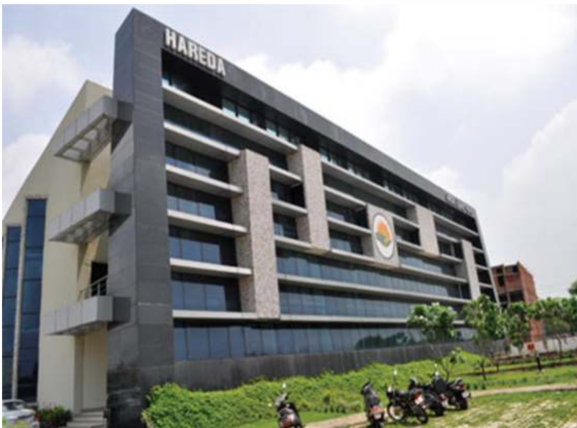
Figure 6: Building of HAREDA
