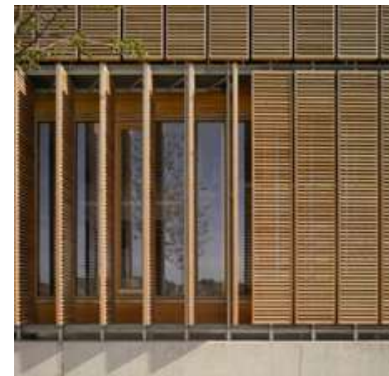
FIGURE 26 AUTOMATED SHADING SYSTEMS
