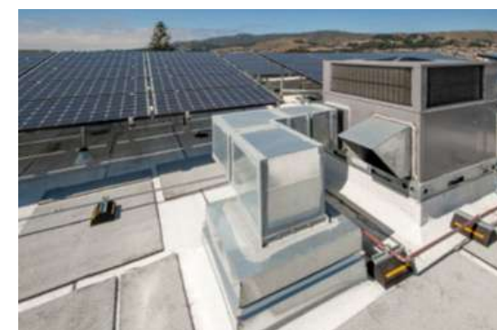
FIGURE 31 INSTALLING HIGH-EFFICIENT HVAC SYSTEM
