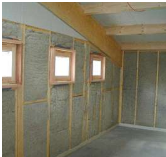
FIGURE 15 WALL AND ROOF INSULATION MATERIAL
