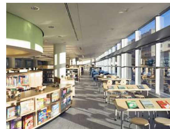
FIGURE 14 INTERNAL AND EXTERNAL LIGHT SHELF
