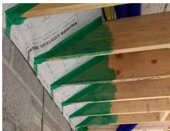
Targeted air sealing defines air barrier
