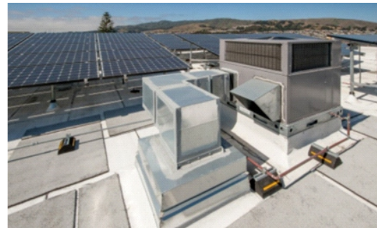
FIGURE 28 INSTALLING HIGH-EFFICIENT HVAC SYSTEM
