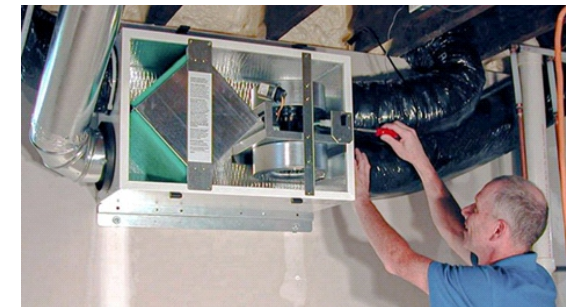
FIGURE 26 ENERGY RECOVERY VENTILATION (ERV) SYSTEMS
