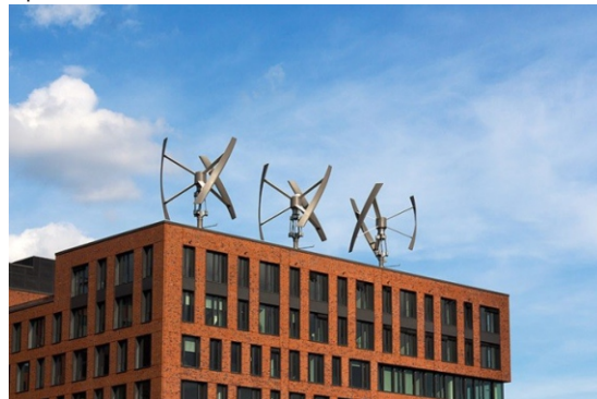
FIGURE 49 ROOF TOP WIND TURBINE
