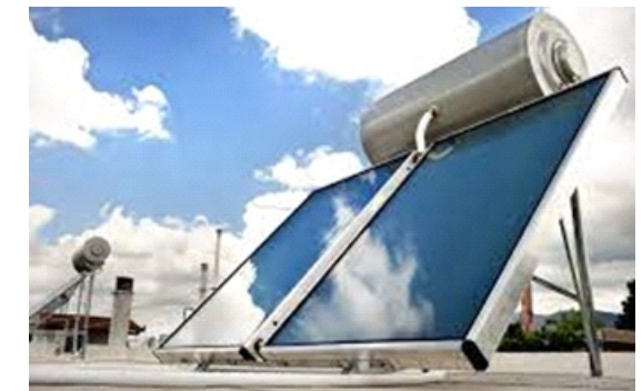
FIGURE 36 SOLAR WATER HEATER
