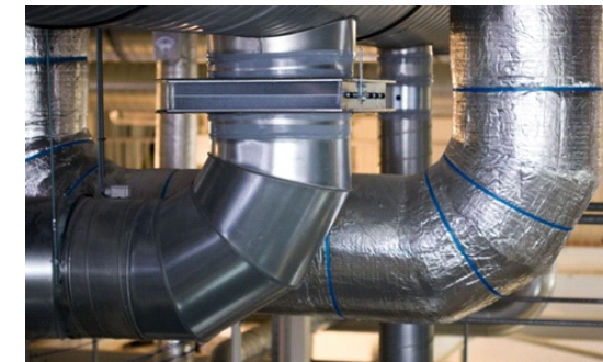
FIGURE 25 SEALING OF DUCT
