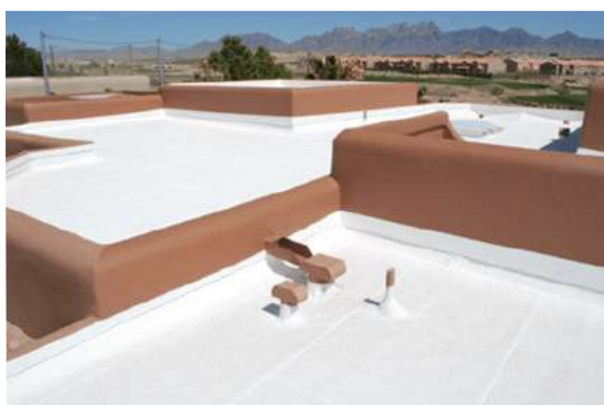
FIGURE 5 HIGH SRI PAINTS ON ROOF
