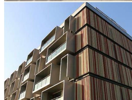
FIGURE 12 EXTERNAL SHADING DEVICES
