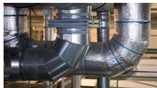
FIGURE 36 SEALING OF DUCT
