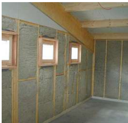
FIGURE 14 WALL AND ROOF INSULATION MATERIAL
