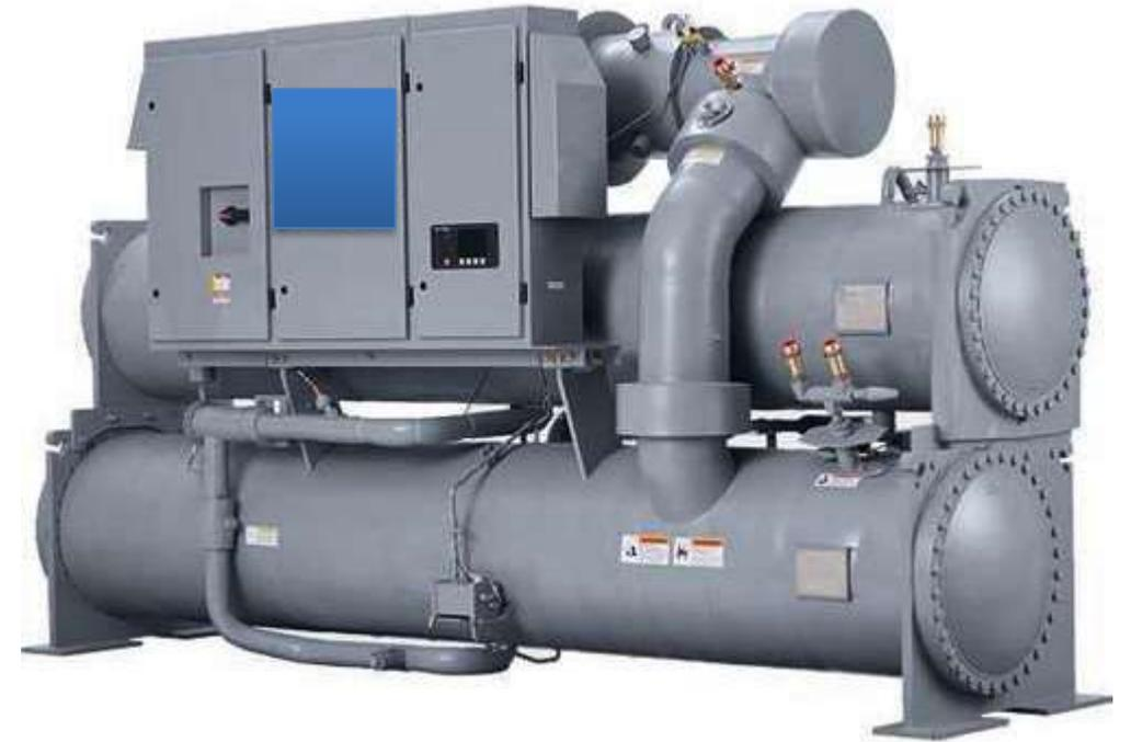
*Fig. water cooled Chiller*
