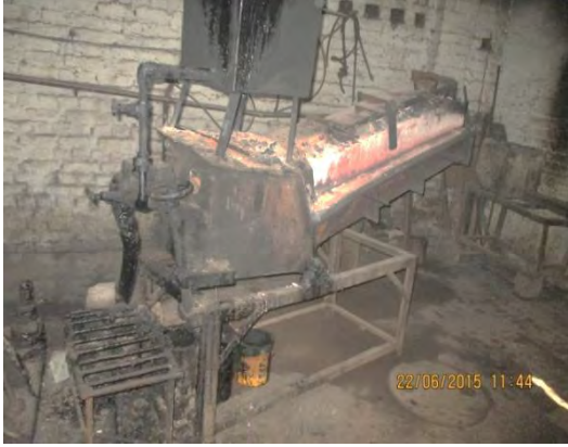
Figure 2.3: Snap shot of FO based re-heating furnace at Allied engineers
