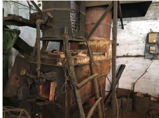
Figure 2.1: Oil fired re-heating furnace (Presently dismantled)
