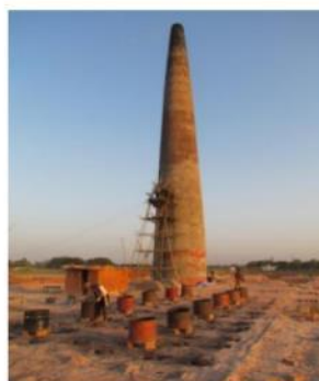
Photo showing longer coal feeding zone
