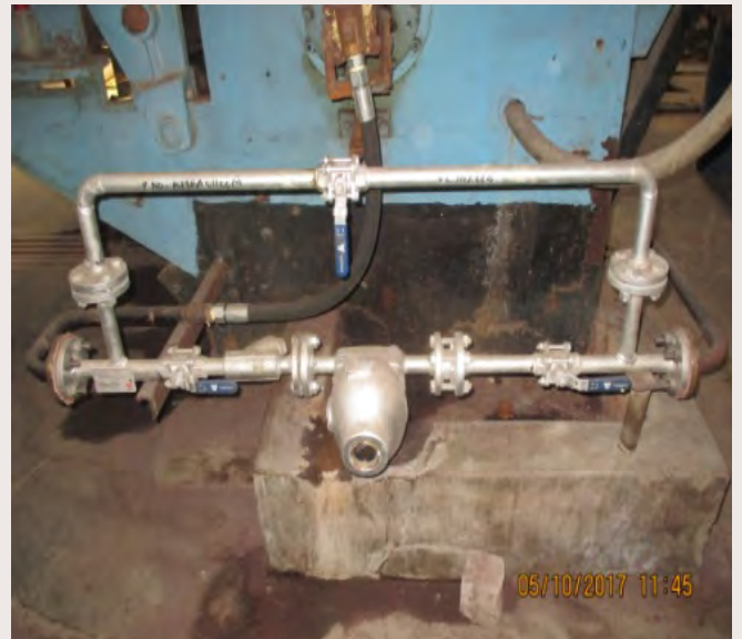
Float trap installed at Rajaram Mills
