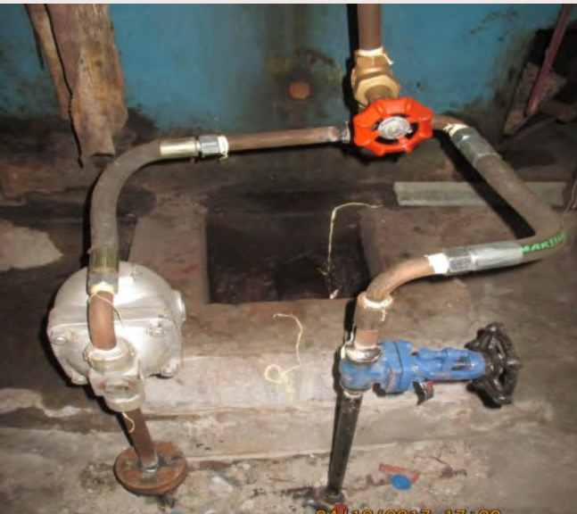
Float trap installed at Simandhar Fabtex
