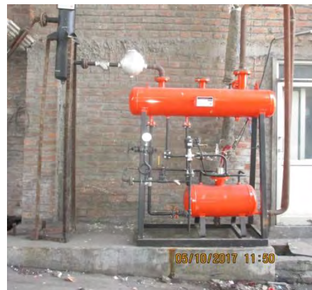
Snap shot of zero-zero machine with condensate recovery system at Shree Rajaram Mills
