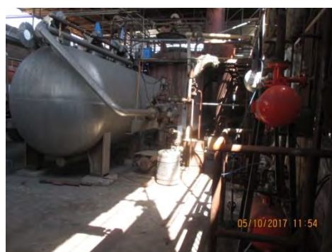
Snap shot of kier boiler with condensate recovery system at Shree Rajaram Mills
