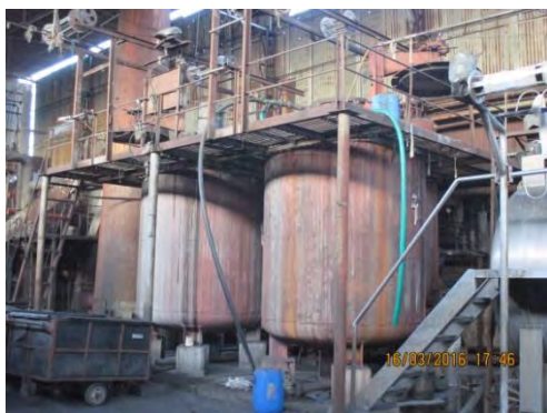
Snap shot of kier boiler without float trap at Shree Rajaram Mills
