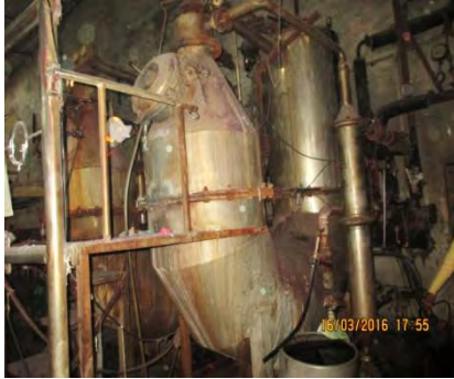
Snap shot of Jet dyeing without condensate recovery system at Shree Rajaram Mills
