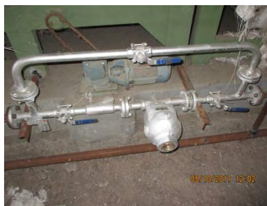
Snap shot of zero zero machine with float trap at Shree Rajaram Mills
