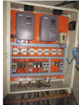
Snap shot of boiler with VFD at Shree Rajaram Mills
