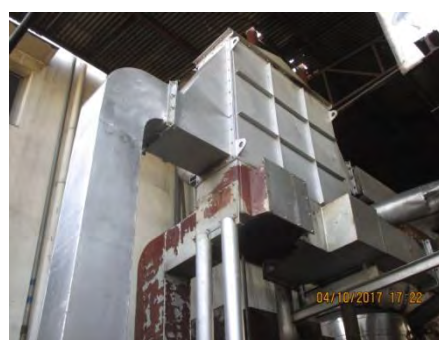
Snap shot of boiler with air preheater at Simandhar Fabtex (P) Ltd
