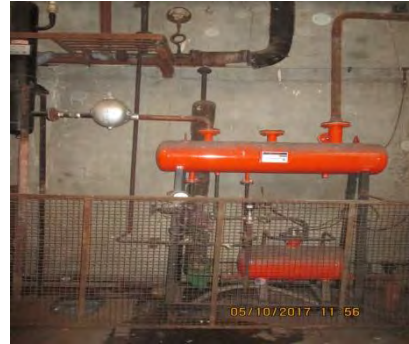
Snap shot of Jet dyeing with condensate recovery system at Shree Rajaram Mills
