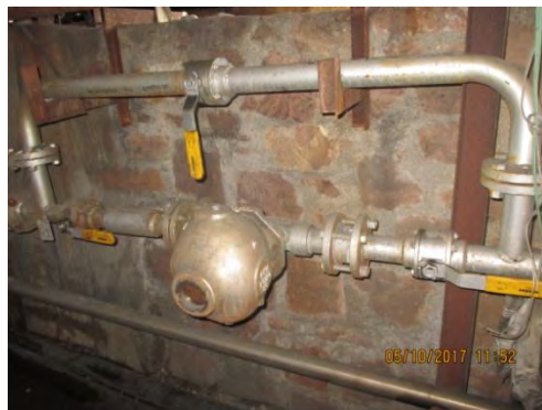
Snap shot of kier boiler with float trap at Shree Rajaram Mills
