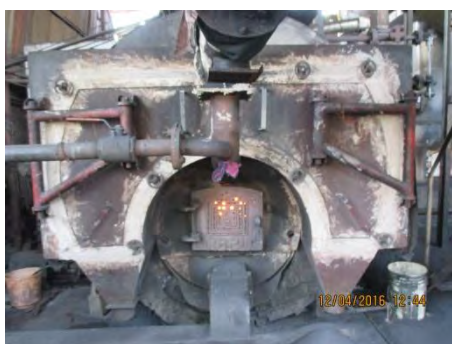
Snap shot of boiler without air preheater at Simandhar Fabtex (P) Ltd
