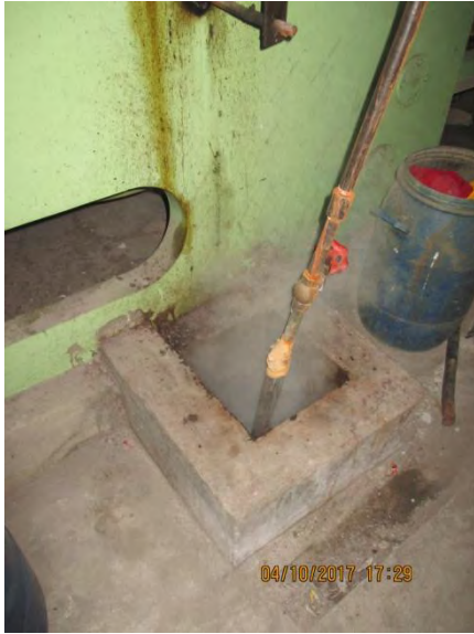
Snap shot of zero zero machine without float trap at Simandhar Fabtex (P) Ltd
