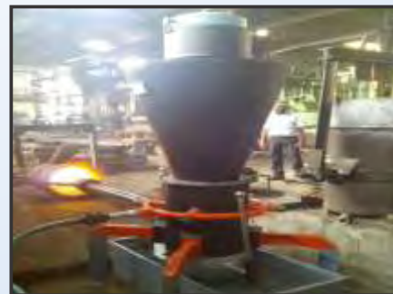
Installation of Biomass Gasifier for ladle preheating process
