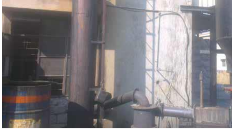
Figure 50 Biomass Gasifier installation
