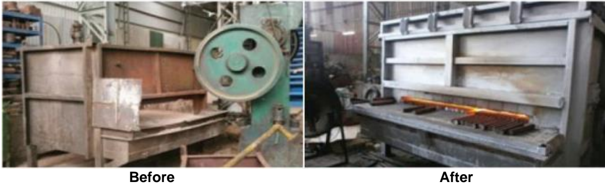
Figure 27: Application of ceramic fibre insulation on hot surface
