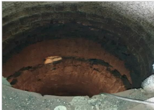
Before: Charge height in stack not maintained
