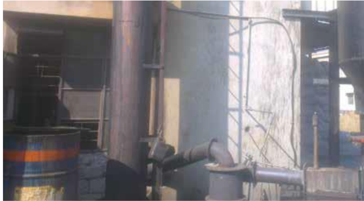
Figure 75 Biomass Gasifier installation
