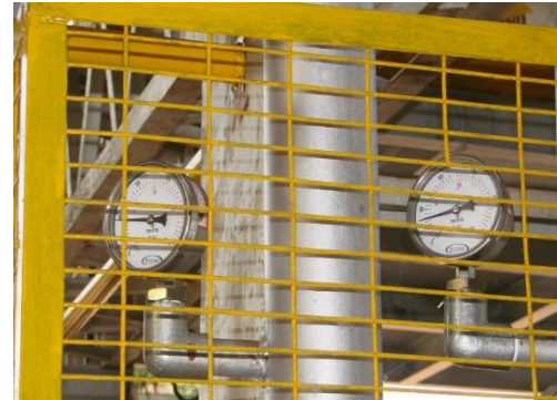
After: Install gauge in accessible location
