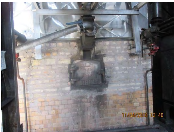
Boiler heating chamber
