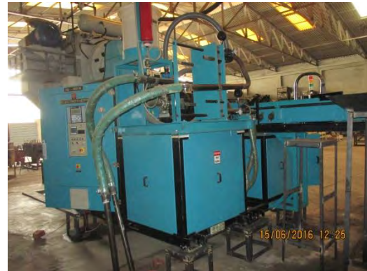
Induction heater installed at Global Exports India
