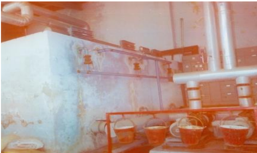
Ice built tank
