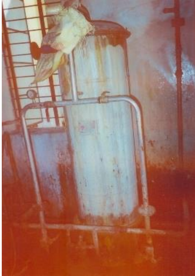
Water filter for boiler
