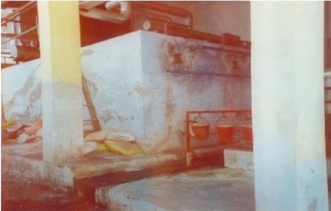
Ice built tank
