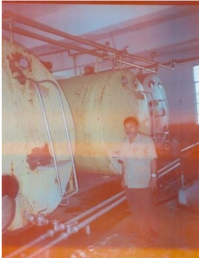
Chilled milk tanks with insulated covered
