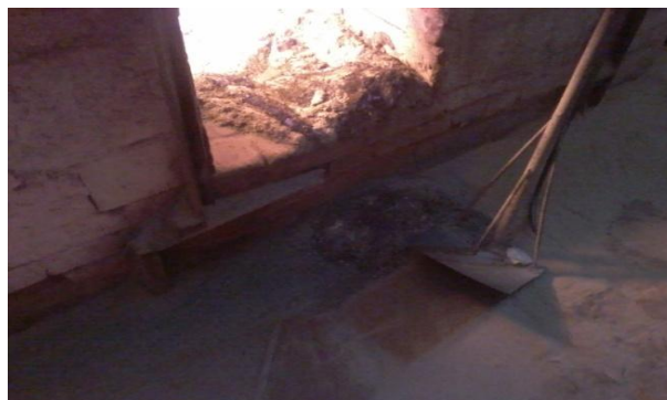
Figure 13: Ash removal opening in roaster
