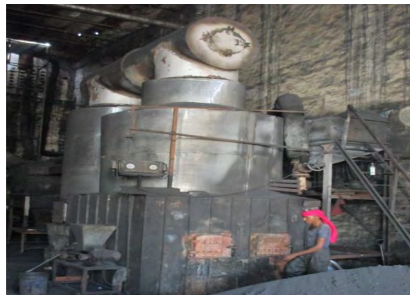
Caption: Thermo-fluid boiler unit at KB Dyeing
