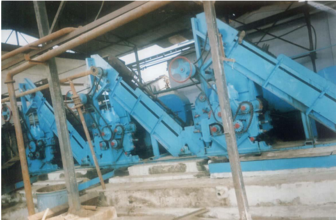
Part of crushing machine
