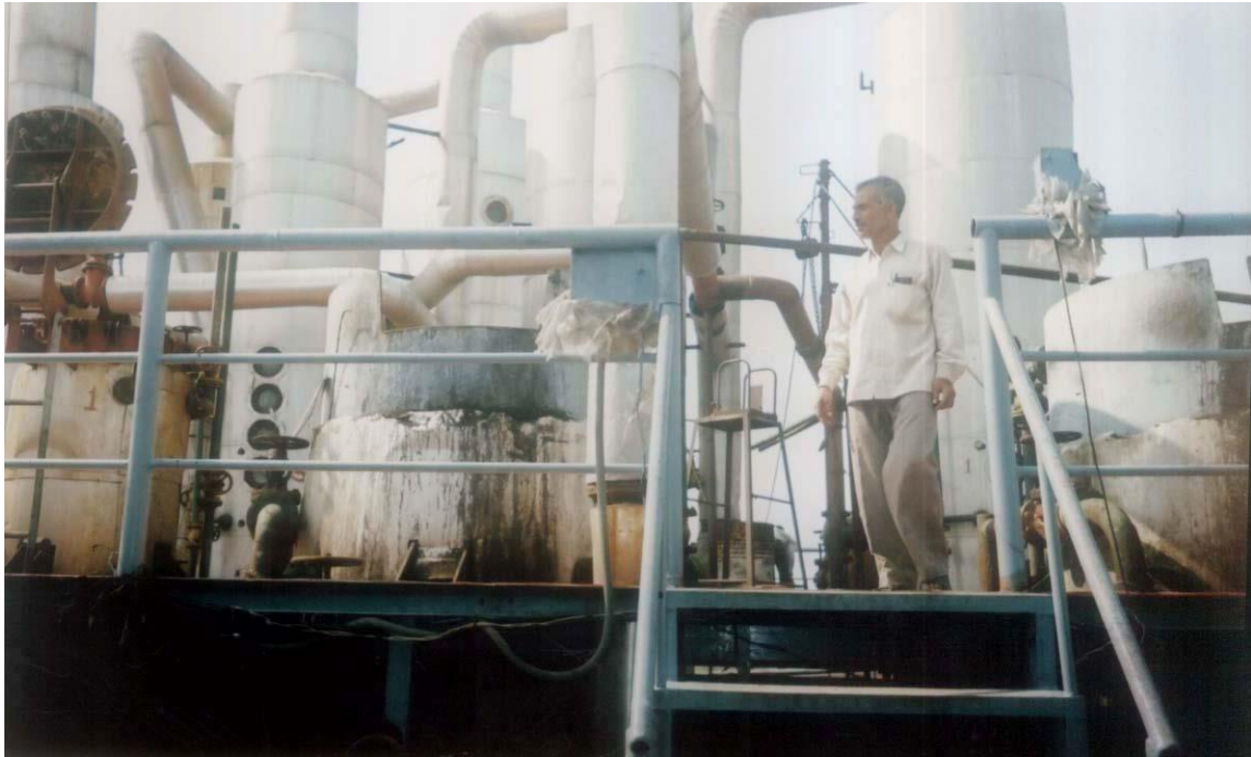
Boiling & crystallizer plant
