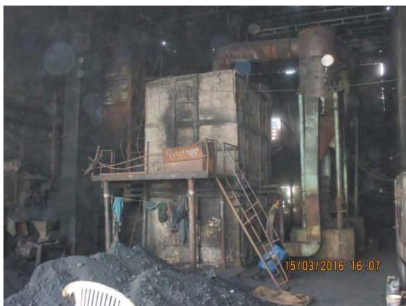
Caption: Boiler unit at Manoj Dyeing
