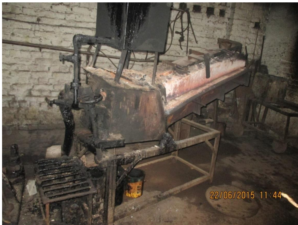
Conventional oil fired burner being used in the unit
