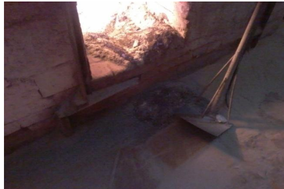
Figure 13: Ash removal opening in roaster
