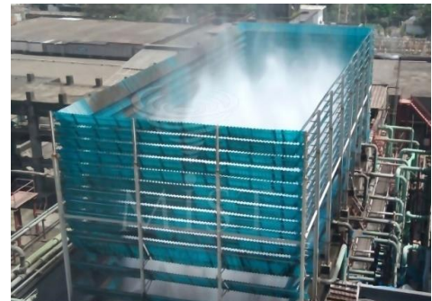
Mist Cooling System for Cooling
