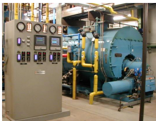
Figure 73: Oxygen trim system connected to boiler
