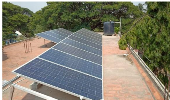
Figure 76: Rooftop solar PV system
