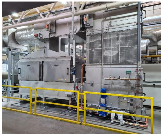
Figure 63: Waste heat recovery system with integrated exhaust air filter system
