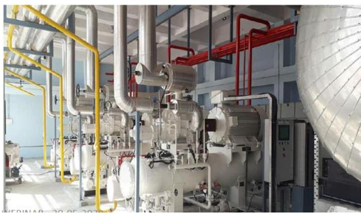
The screw compressors with VFD have low specific energy consumption compared to reciprocating compressors resulting in low energy consumption for refrigeration purposes. Reciprocating compressors often face load cut-off issues when the demand fluctuates, whereas screw compressors adapt smoothly to varying loads. They offer the advantage of facilitating gentle startup and shutdown procedures, even when operating at maximum load capacity.
