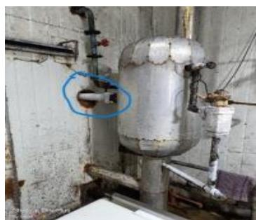
*Figure 48: Accumulator pipe*
