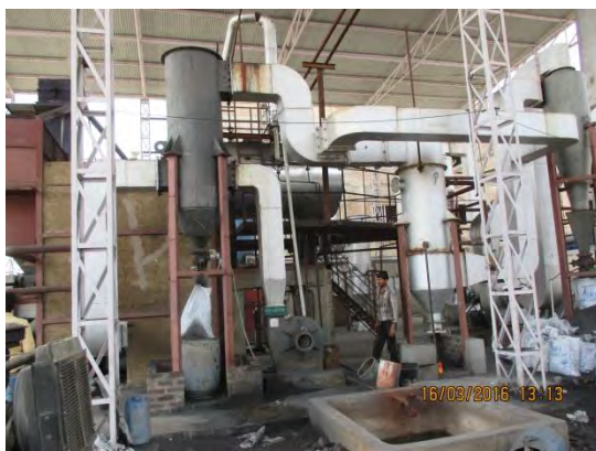
Caption: Boiler unit at Shree Rajaram Prints (P) Ltd.
