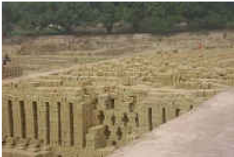
Image 4: Wet Green Brick drying
