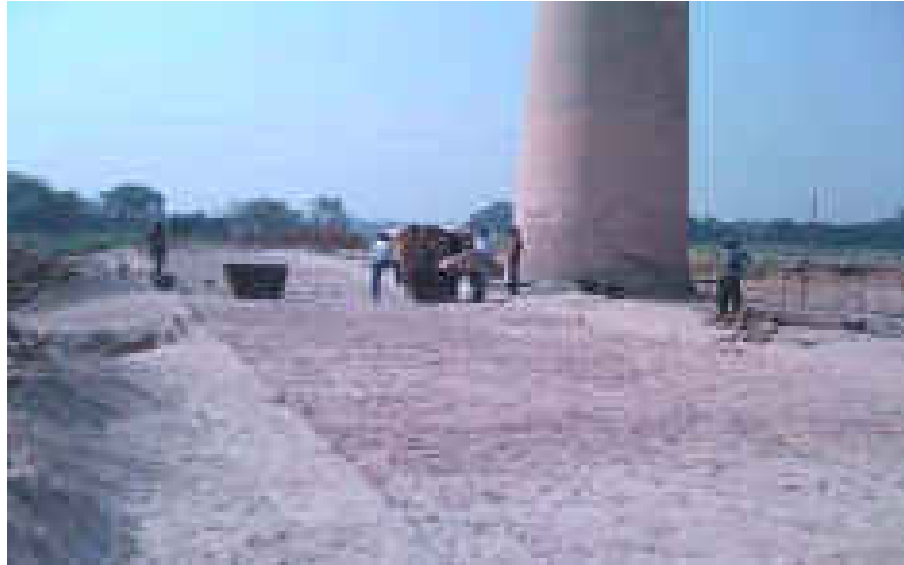
Image 2: Traditional Fixed Chimney BTK
