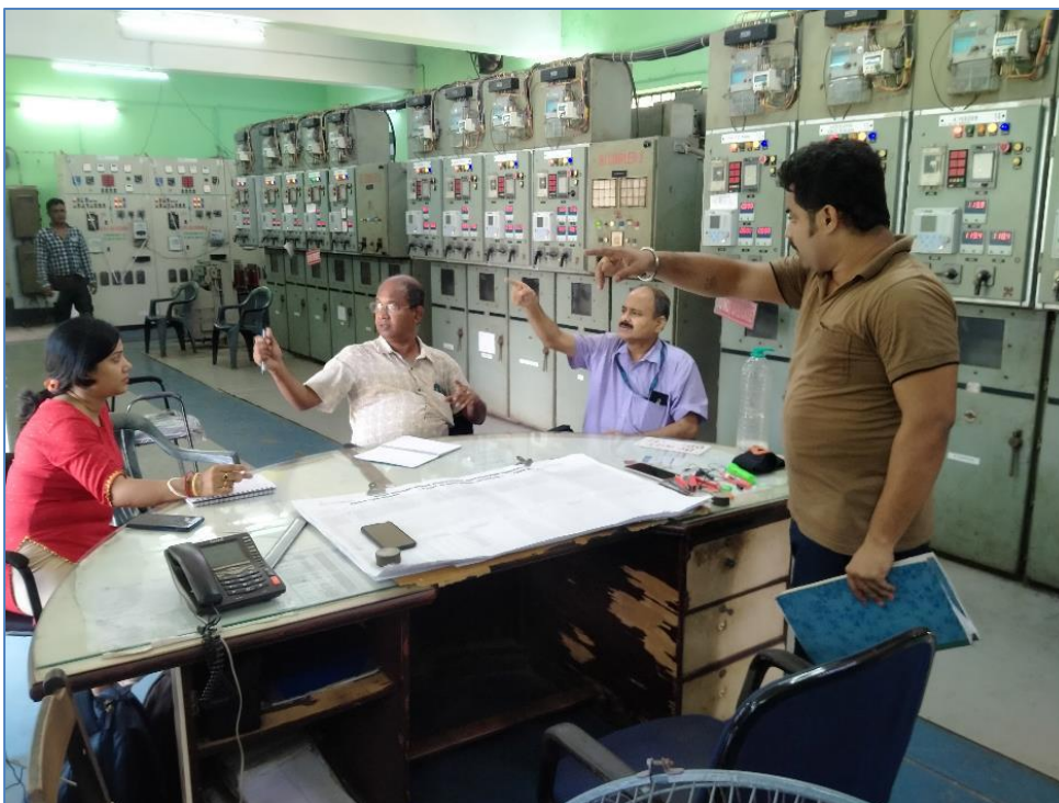
Figure: Discussion with Engineer at M-III Substation
